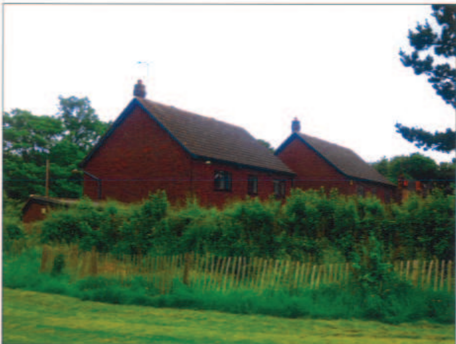
Fron Cottage viewed from recreation ground (Farm Cottage in foreground)
